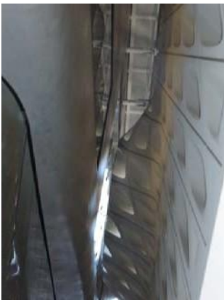
Detail of the concrete wall and fiber reinforced concrete facade.
