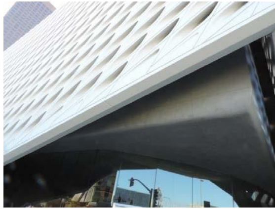
Detail of the concrete wall and fiber reinforced concrete facade.
