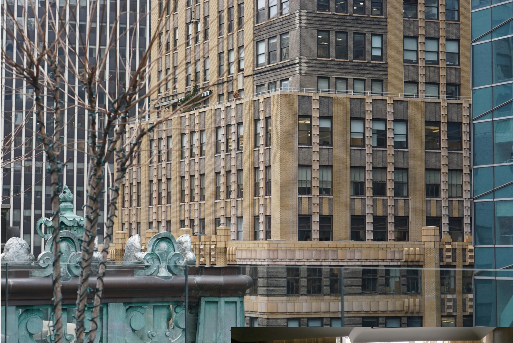
Beaux-Arts façade building :
