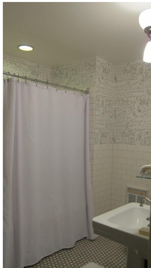
Shower Area behind Curtain :
